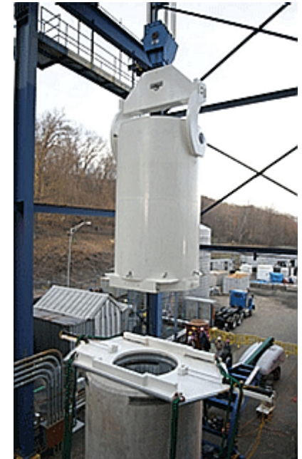
Placement of a multi-purpose canister at a NAC project
