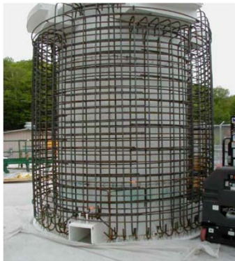
Canister under construction at NAC Project Site
